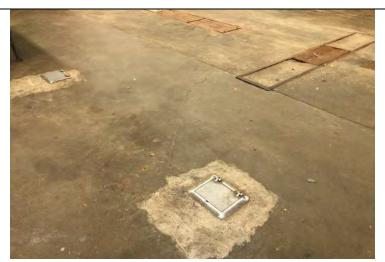
Photo 13: Inactive in-ground lift in automotive shop.
