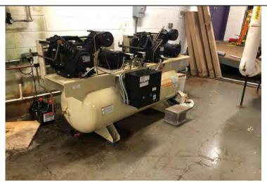
Photo 2: Air compressor in the main building boiler room.
