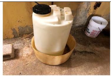
Photo 24: Muriatic acid tank in pool mechanical room. Tank in secondary containment.
