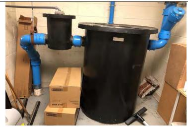
Photo 29: Waste acid tank for used classroom chemicals. Located on the first floor near classrooms numbered in the 500s.
