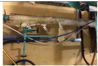
Photo 19: Pipe wrap in pool mechanical room
