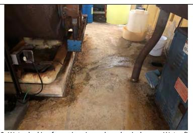
Photo 20: Water leaking from pipes in pool mechanical room. Water flowing into a floor drain.
