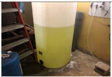
Photo 22: Leaking chlorine tank in pool mechanical room.
