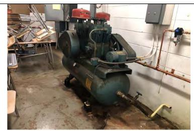
Photo 4: Air compressor in main building boiler room.
