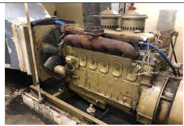
Photo 7: Diesel-fueled generator in main building.
