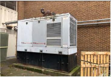
Photo 30: 500-gallon diesel-fueled generator located in the northern portion of the site. Used to power the fire pump system.
