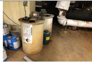
Photo 9: Two containers of Biosperse 254 microbiocide next to old chiller in main building.
