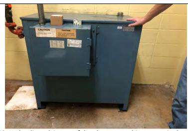
Photo 39: Hydraulic tank in one of the elevator machine rooms in the main building.
