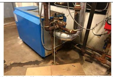
Photo 48: Boiler in the old vocational agricultural building. Visible staining on the ground.
