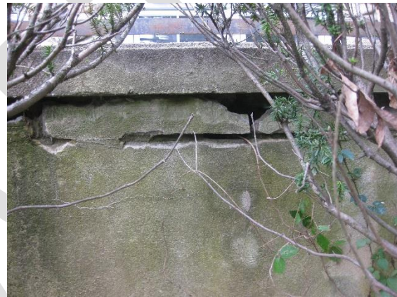
#26 – Cracks and voids below ramp slab
