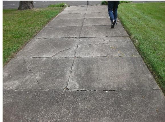
#24 – Cracks at spalls at front walk
