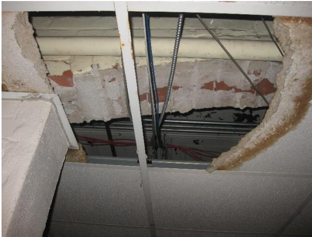
#13 – Brick arch at interior bearing wall
