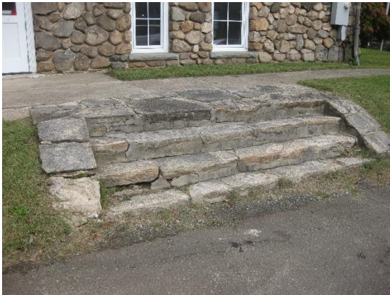
#23 – Cracks at south side stairs
