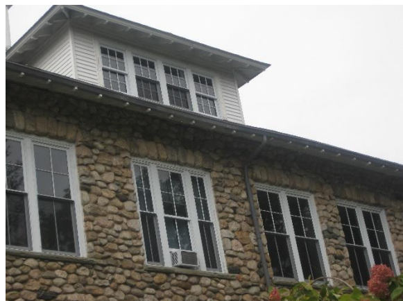
#16 – Sagging gutter above front entrance
