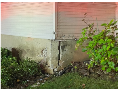
Speeding car blew through stop sign at Hubbard and Bridge and plowed into a house on the corner, cracking the cement foundation, destabilizing the home.
