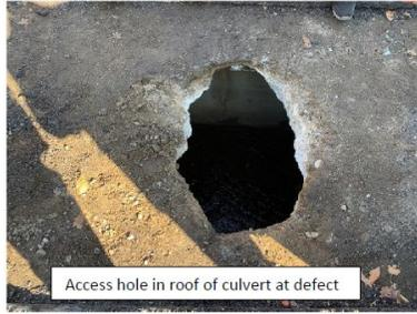
Access hole in roof of culvert at defect
