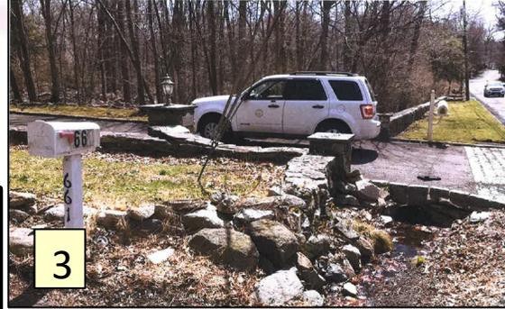
@ Driveway apron to 655 West Hill Rd. Sinkhole opened up @ corr. Metal storm pipe within ROW
