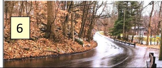
4/2/2019 @ 661 West Hill Rd. Note condition of deteriorated road and storm piping under driveway to 655 West Hill Rd. @ sink hole.
