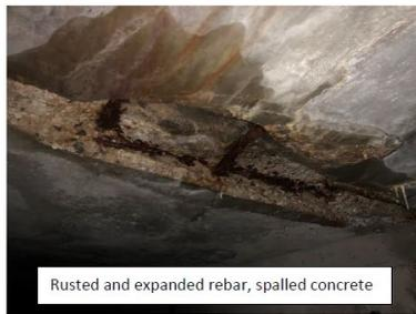
Rusted and expanded rebar, spalled concrete
