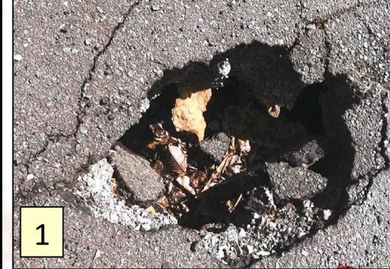
4/2/2019 @ Driveway apron to 655 West Hill Rd. Note condition of deteriorated road and sinkhole @ 655 West Hill
