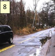
12/14/2020 @ 643 West Hill Rd. looking south toward MacGregor Dr. Note puddle @ right side of road. Believe this portion of roadway previously drained into the stream on west side of roadway, and is currently not properly draining due to construction of asphalt curb and walkway on west side of road, which obstructs previous flow. No drainage
