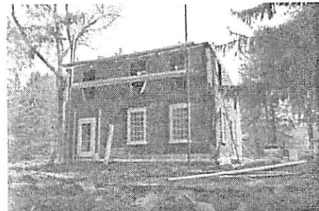
8-12 Free Street, during dismantling
