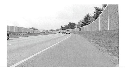
Because noise travels in waves, not straight lines, sounds can and do go over the walls. This is why even with barriers standing 16 feet, homes several blocks away can hear the highway.
