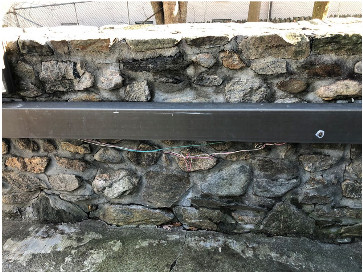
Exposed wiring in ramp handrail
