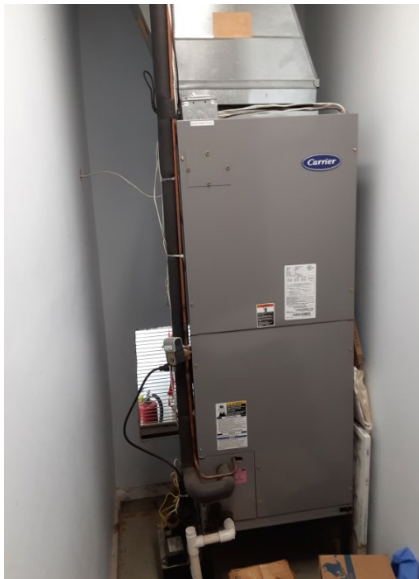
Typical 2 nd Floor Closet Mounted Air Handling Unit
