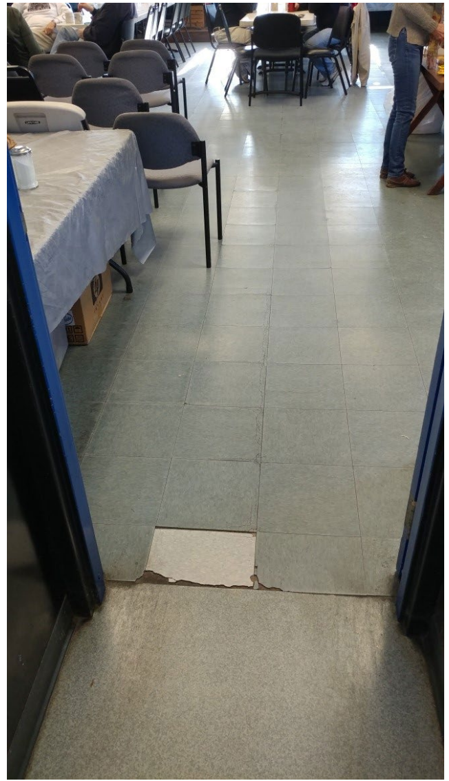
CHIPPED AND DAMAGED FLOOR TILES
