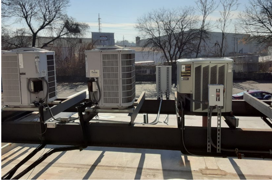
Exterior Condensing Units Located above Restrooms
