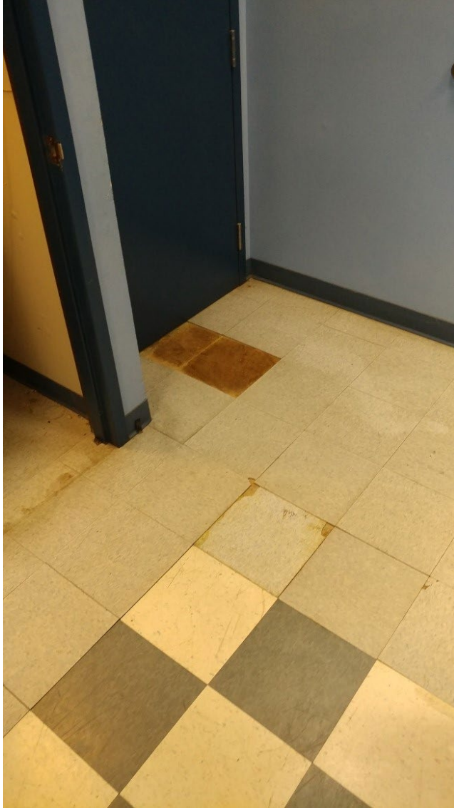
CHIPPED AND DAMAGED FLOOR TILES
