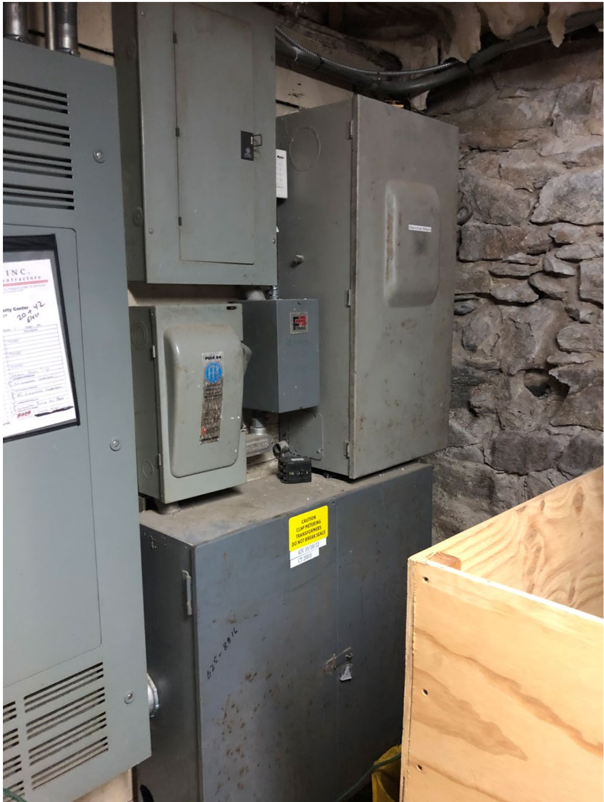
Main Electric Service Entrance in Electrical/Mechanical Room
