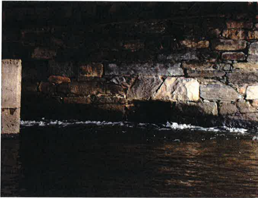
Photo #5 - Main Pier (West Elevation) - Note Approx. 3' Wide by 2' High by 2' Deep Void
