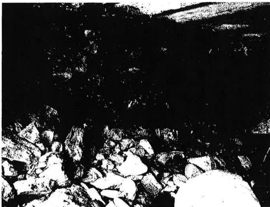
Photo #3 – West Abutment- Closer View of About 22' Wide by 7' High by 6' Deep Void
