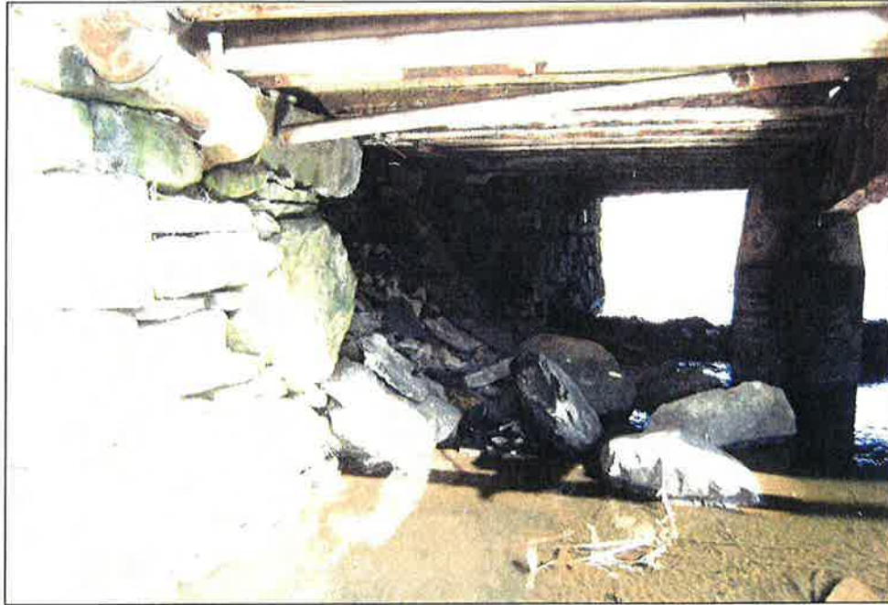
Photo #5 – West Abutment Failure From Downstream
