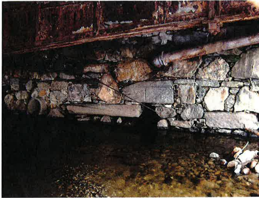
Photo #7 – East Abutment - Note Approx. 2' Wide by 3' High by 6' Deep Void
