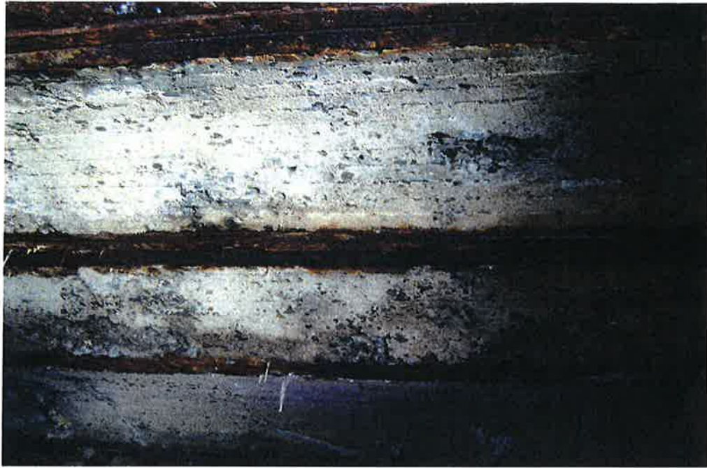
Photo #3 – Typical Underside of East Span – Note Rusting Stringers
