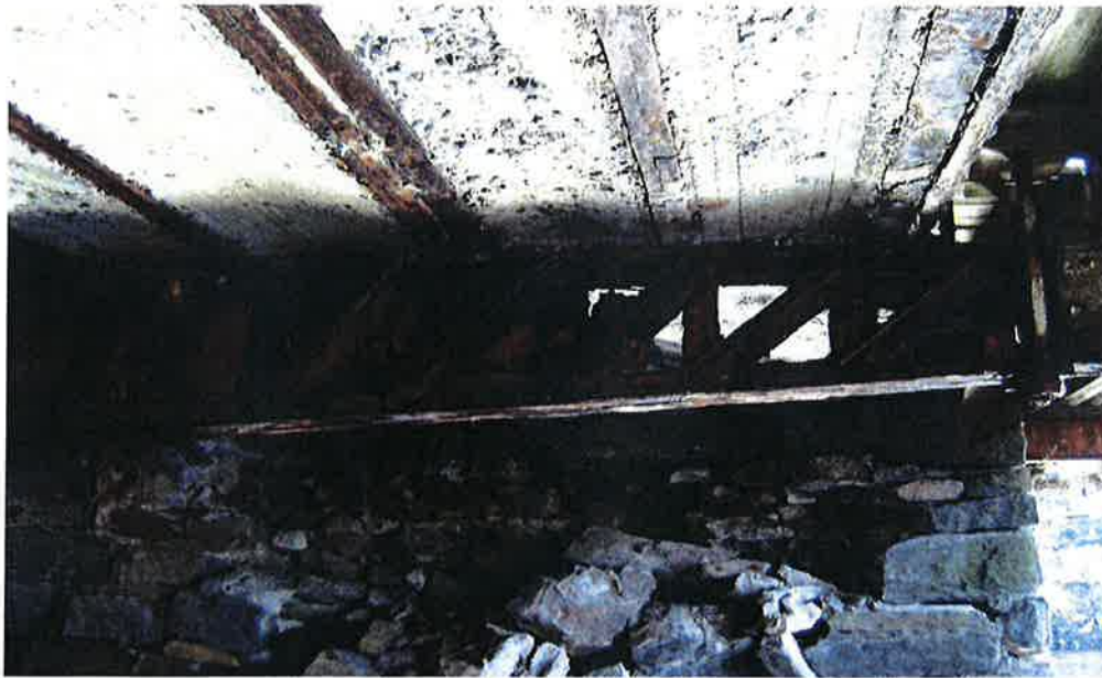
Photo #4 – Typical Underside of West Span – Note Poor Floor Beam Condition
