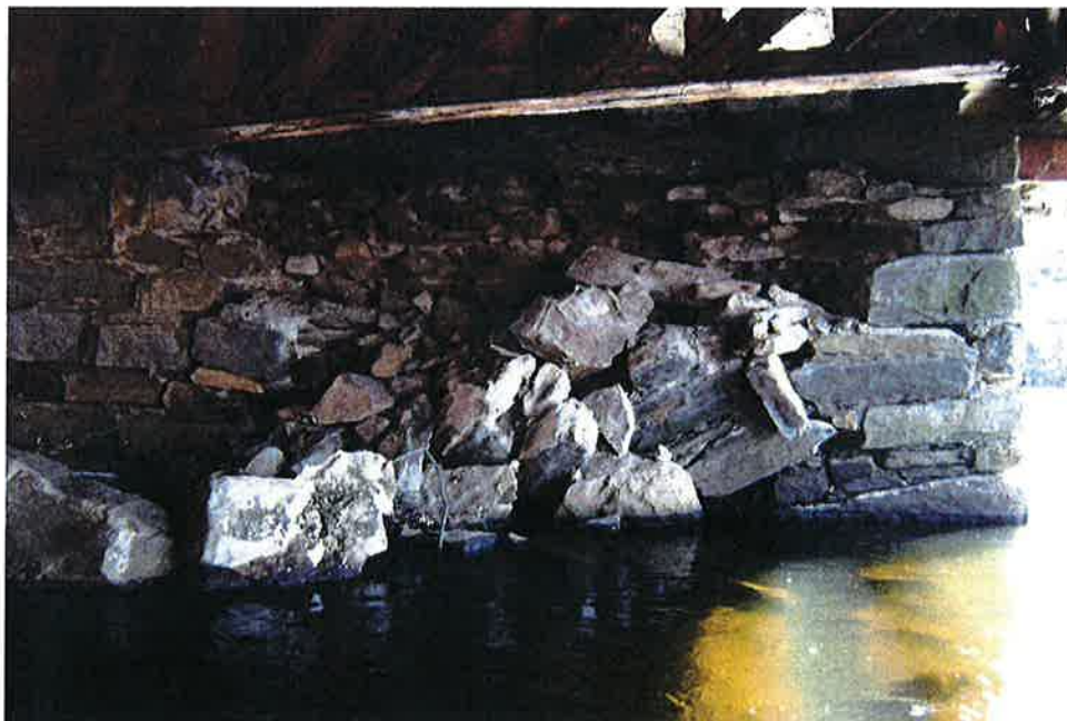
Photo #8 – Close-Up Main Pier Collapse. Also note Hole in Floor Beam.
