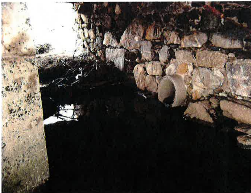
Photo #8 – East Abutment - Note Large Amount of Debris Just Upstream
