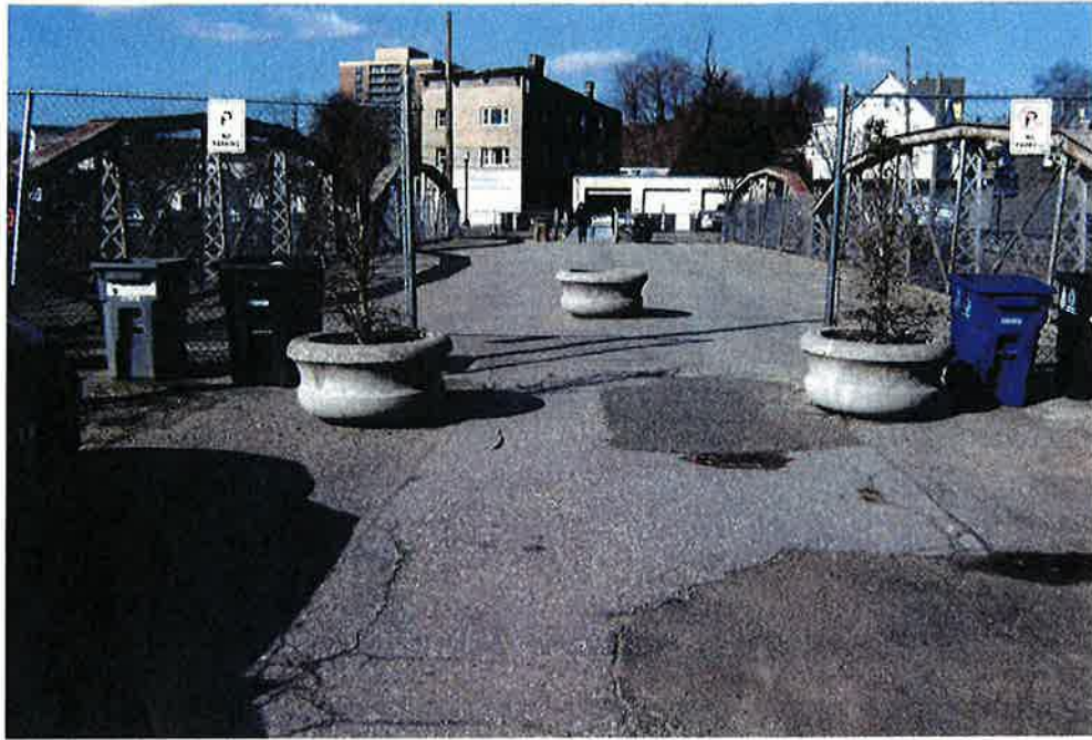
Photo #1 – Bridge Deck Looking West - Note Overall Rusting of Trusses
