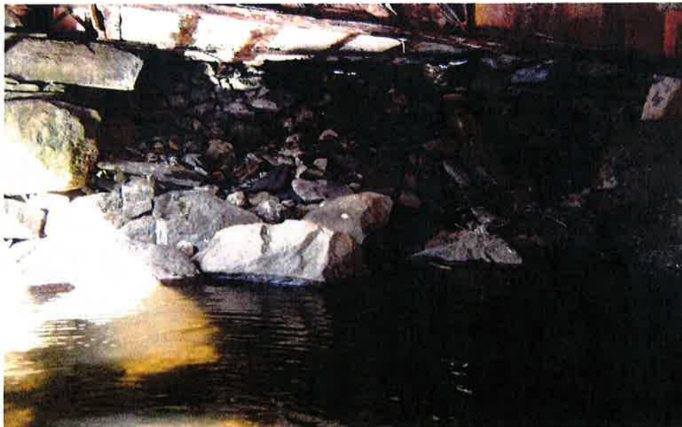
Photo #6 – West Abutment Failure (20' wide x 9' deep x 7' High)
