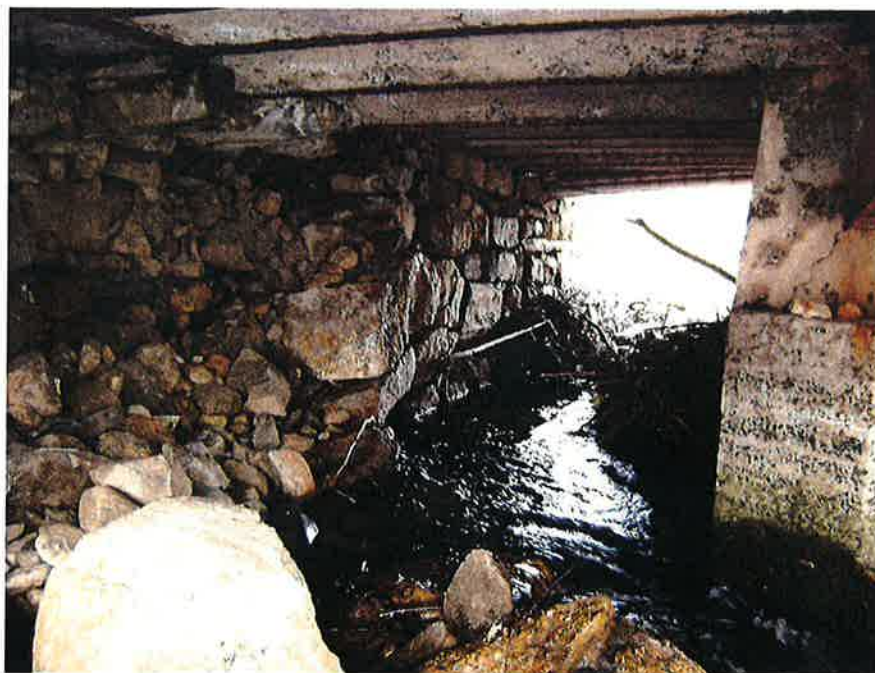
Photo #2 – West Abutment - Note Very Large Void & Large Amount of Debris Upstream
