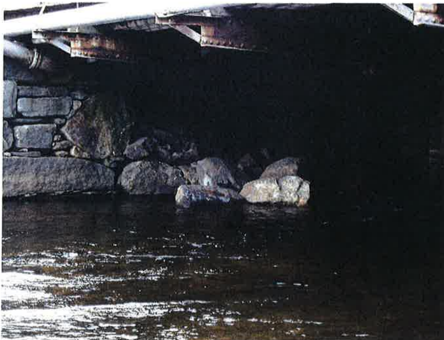
Photo #1 – West Abutment - Note Very Large Void
