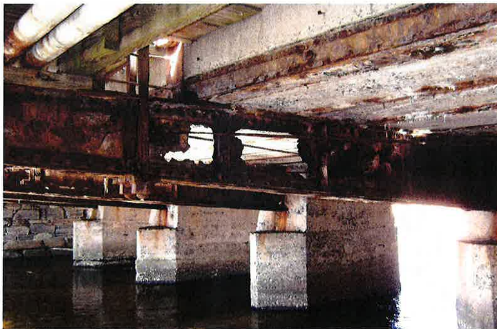
Photo #10 – Close-Up of Deterioration of Downstream East Span Floor Beams.
