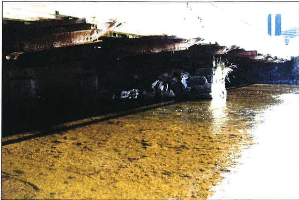
Photo #7 – Main Pier Collapse Downstream End (West Side). Note Floor Beams
