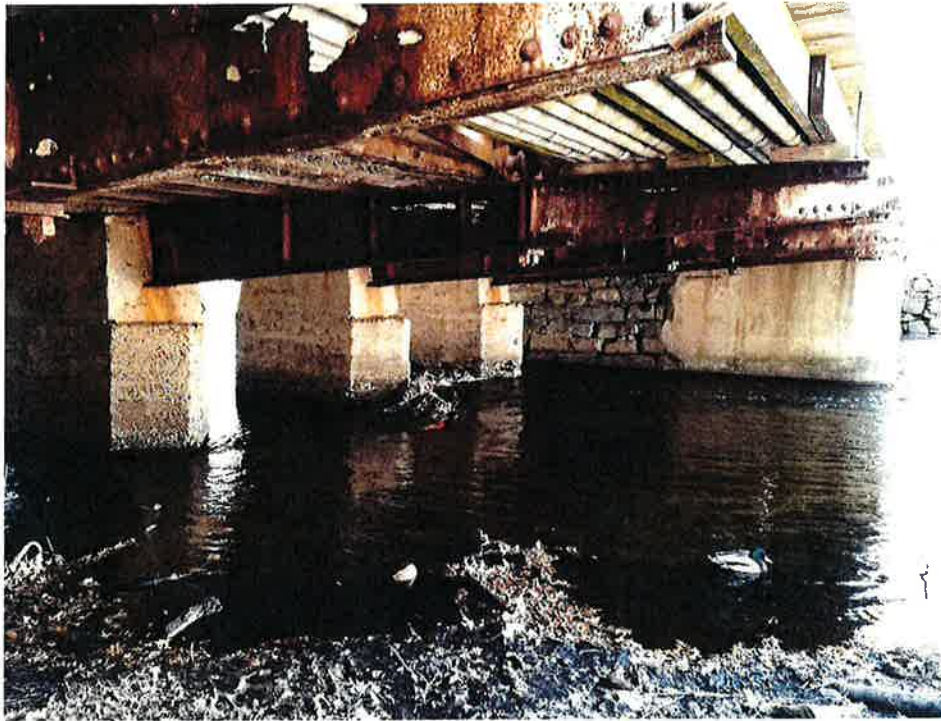
Photo 1: Underside of Bridge showing Floor Beams, Piers, and Utilities (typical)
