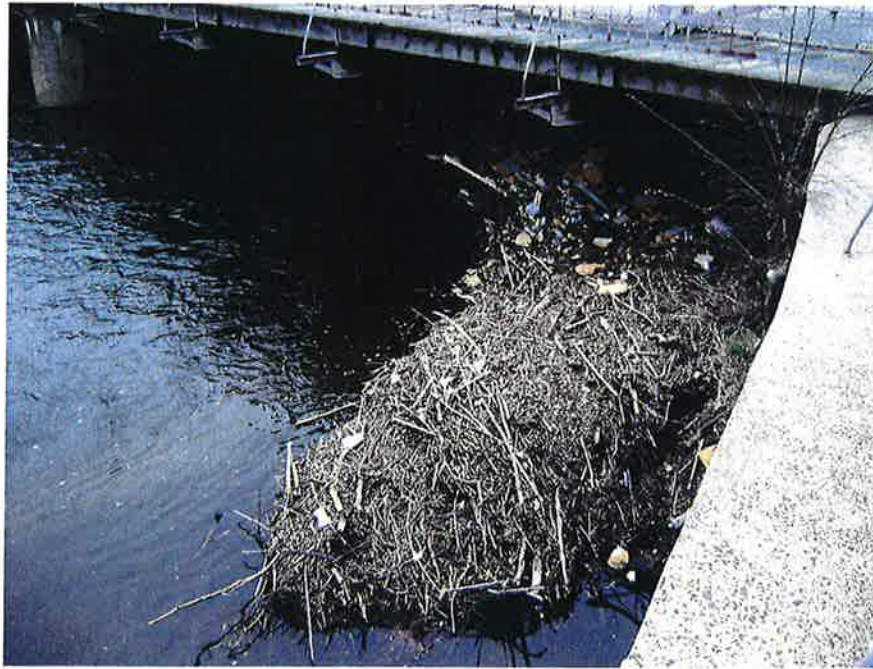
Photo #9 – Upstream of Bridge Near West Abutment - Note Very Large Amounts of Debris
