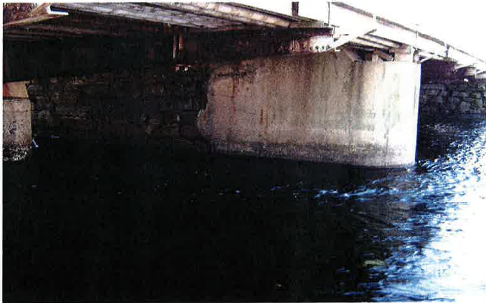
Photo #2 – Upstream End Main Pier – Also Note Rusting & Holes in Floor Beam
