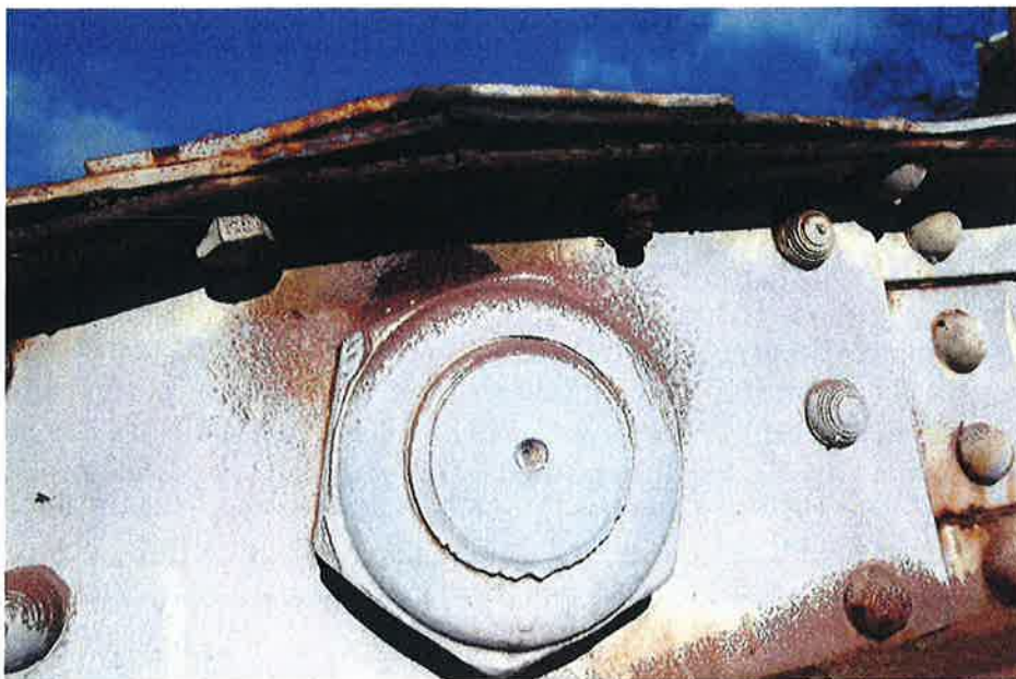
Photo 3: Cover Plate at Lenticular Truss Top Chord Panel Point (Typical)
