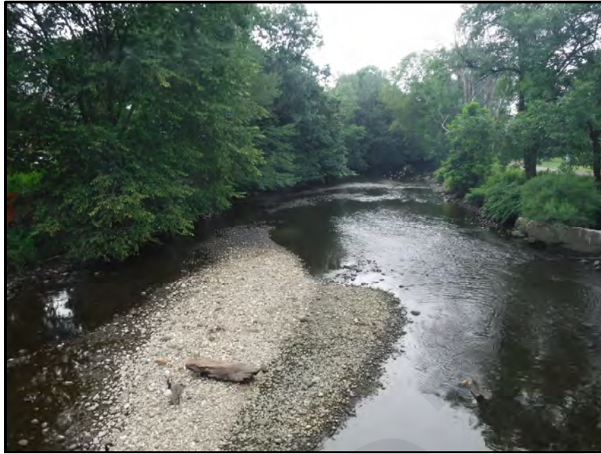
Photo 2: Waterway looking downstream (south).
