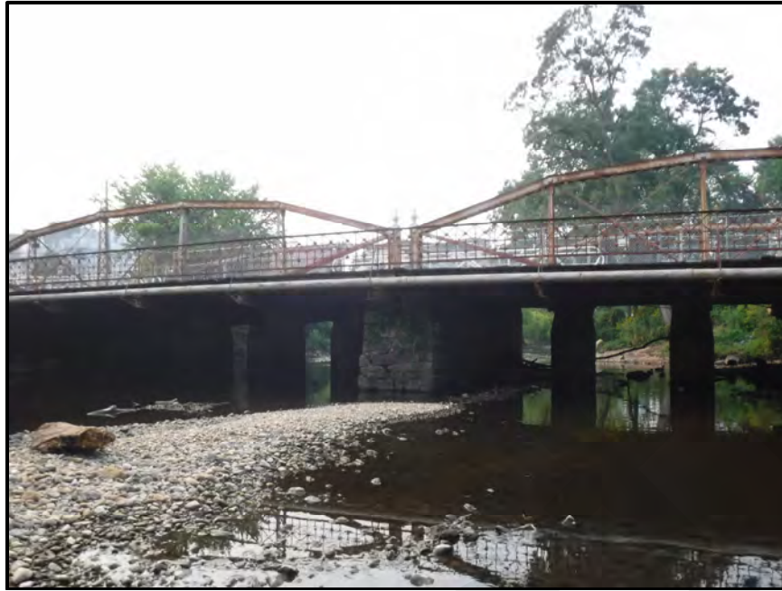
Photo 1: South Elevation of Structure.
