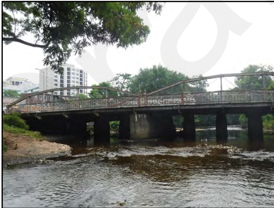
Photo 2: North Elevation of Structure.
