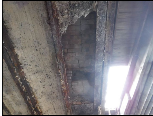
Deck and Floor Beam failure: Looking Up
