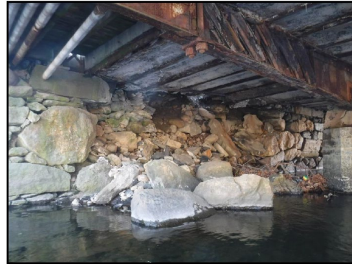
West Abutment and Center Pier Failure
