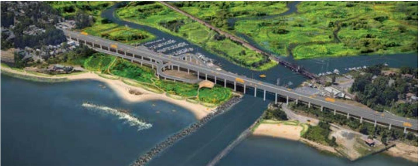
In Cheesequake Inlet, a multi-purpose flood barrier system is integrated into redevelopment sites on either side of Noe's Creek with living shorelines as a buffer.
