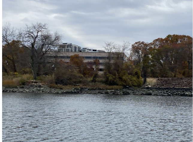
View toward Kosciuszko Park Potential Boat Launch Site 1 nearby Stamford Hurricane Barrier to right. (G. Steadman photo 2025)
