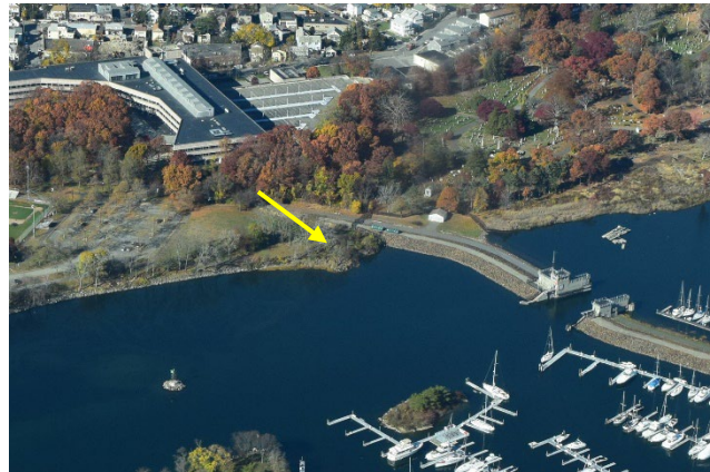
View toward Kosciuszko Park Potential Boat Launch Site 1 nearby Stamford Hurricane Barrier to right. (G. Steadman photo 2016)
